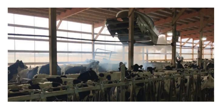
This unique adjustable barn fan is designed so that the louvers give off a laminar flow. That means the airflow can move around the cow in layers of air. Thus, even when your cow is behind a cow or object, it is cooled at all times. A unique system that, among other things, effectively prevents heat stress!
